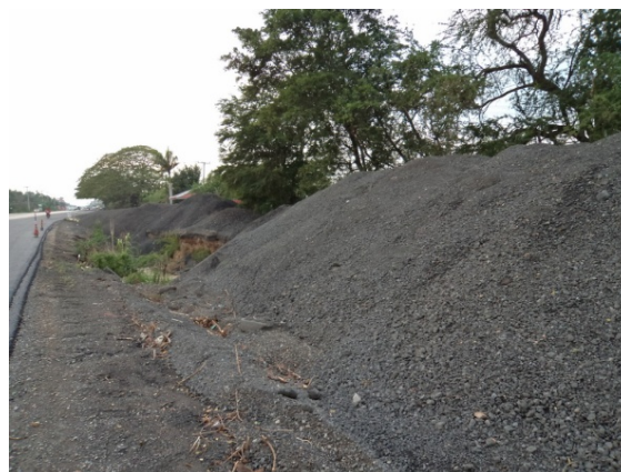
Fig. 1 On-site RAP heap in the Lopburi province, Thailand (photo by Jirayut Suebsuk)
