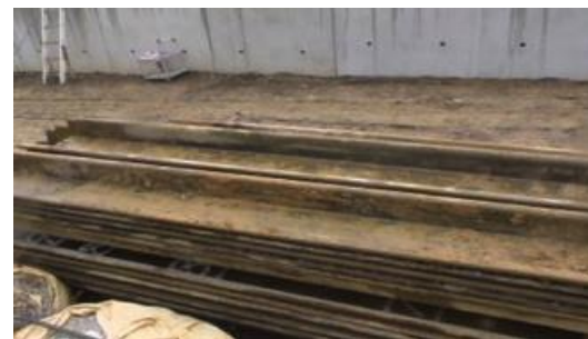
Photo. 6 A steel sheet pile after pulling-out
