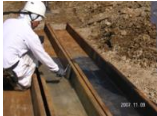
Photo. 4 Working scenery of applying WSFRM to a steel sheet-pile
