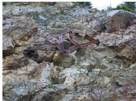
Fig. 4 Rock mass exposure showing the blocky nature of the rock mass
