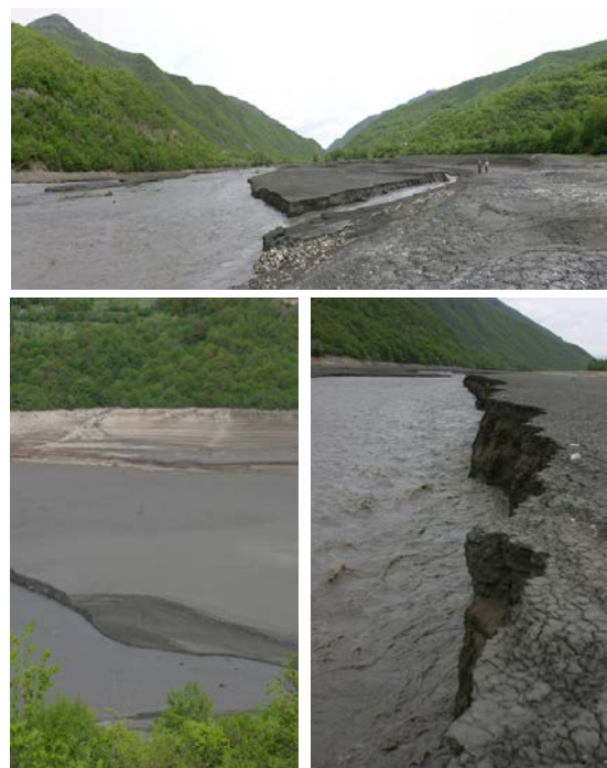
Fig. 3 Silting prism fragments (Jinvali reservoir)
