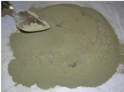
Fig. 4. Mixing MS fibers to Dry Mortar
