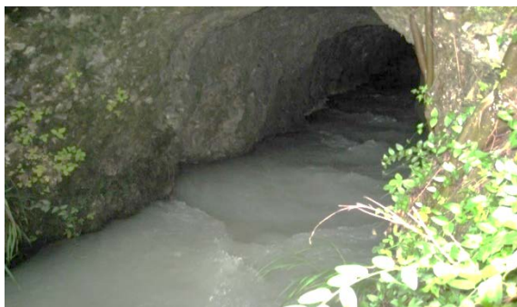
Fig.2 The spring with the highest yield of filtrate in the derivation tunnel
