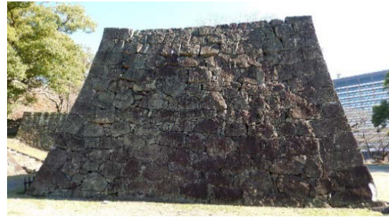
Photo 2 Stonewall of "Chayagura" trace
