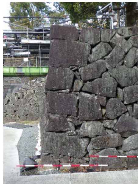
Photo 1 State of pole installation
