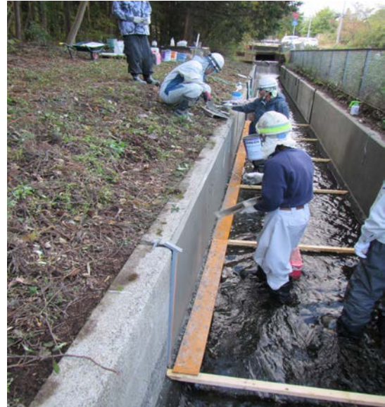
Fig. 1 Workers repairing a deteriorated river canal in Kochi.
