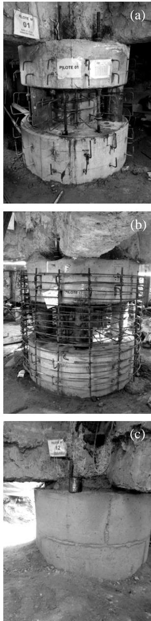
Fig. 8 Reconstruction of piles after the leveling process: (a) Dywidag bars and steel tubes between caps; (b) reinforcement around pile and caps; (c) final condition and soil infill
