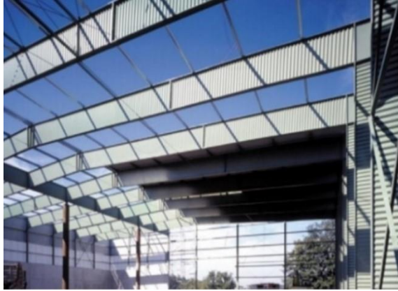
(a) Industrial Building [2]
