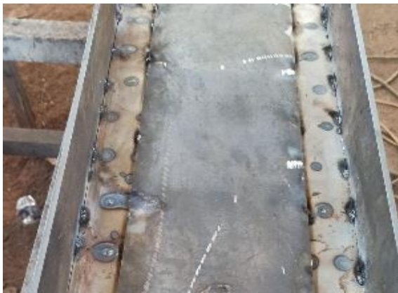
(b) Welding the web to the flanges
