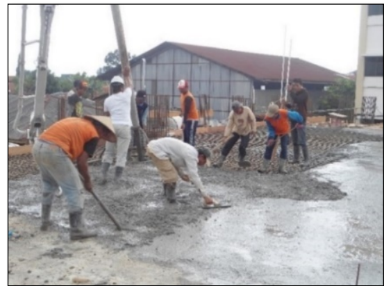
Fig. 2 Casting the concrete of the second-floor plate
