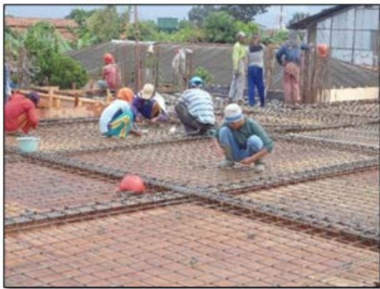
Fig. 1 Putting together the steel reinforcement on the second-floor plate
