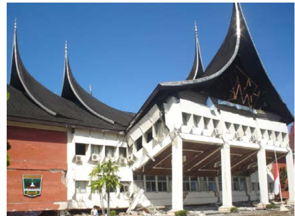
Fig. 7 A typical first soft story in Padang 2009
