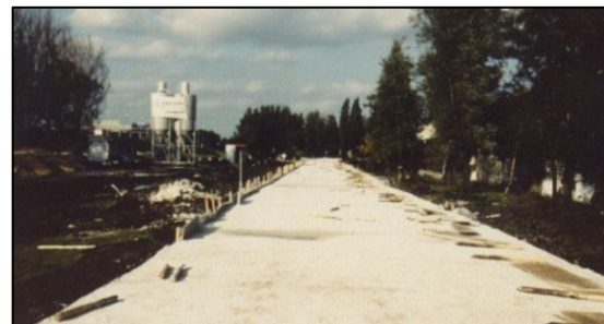
Fig. 1 Concrete raft used as a floating housing road in the Netherlands [15]
