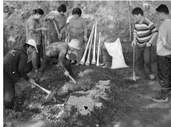
Fig.5 Stabilization treatment of foundation by cement-mixed soil
