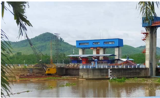
Fig.2 The activity of sediment dredging in Sengguruh Reservoir
