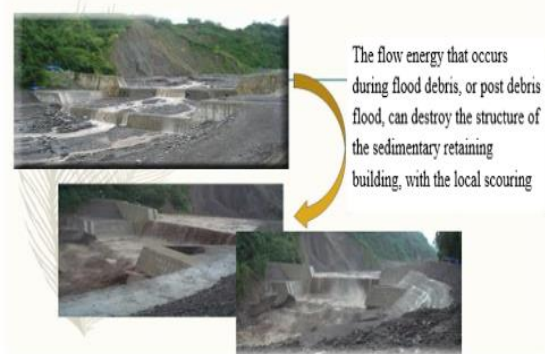
Fig. 1 The process of local scouring on the downstream of sabo dam structures (after Maddi et al., 2018)
