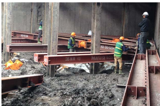
Fig.4 108 Military Central Hospital project constructed the basements by the strut system combined with hydraulic jacks
