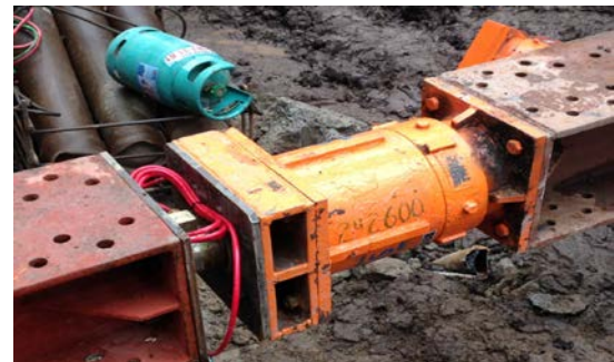
Fig.7 The link between hydraulic jack and steel H-beam
