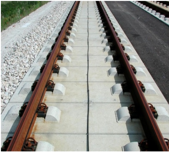
Fig. 1 Typical slab track
