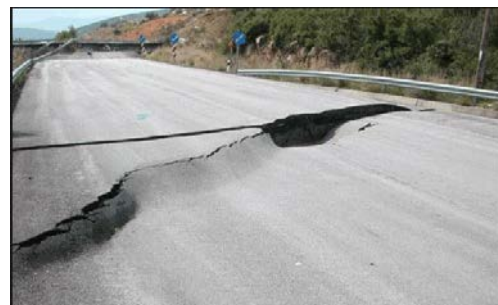
Fig.1 Illustration of the uneven surface due to creep deformation of subgrade, [5]
