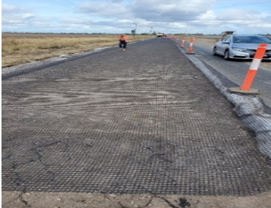
Fig. 9 Placing Foreac 80 MD on Geocomposite
