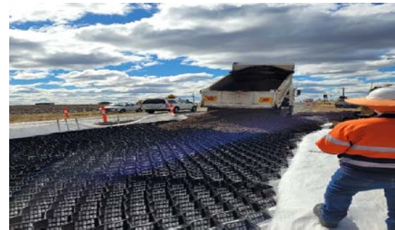
Fig. 7 Placing material and fill voids
