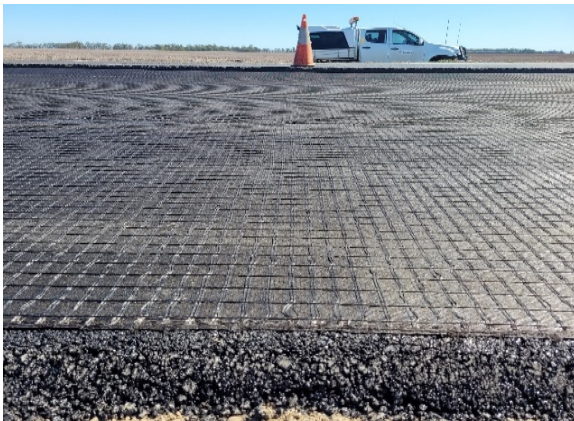
Fig. 10 Placing Geosynthetic Material (Trial 7 and 8)
