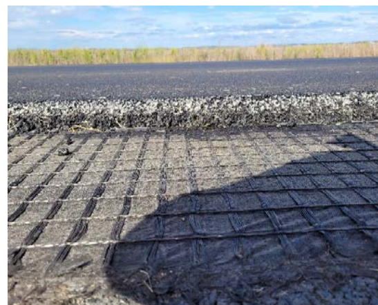
Fig. 3 Trial 1 using Hatelitic C
