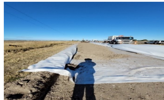
Fig. 8 Placing Geocomposite
