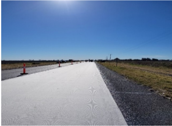
Fig. 4 Geotextile on tack coat
