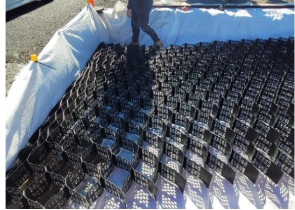
Fig. 6 Placing Geogrids on Geofabric
