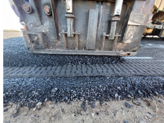
Fig. 11 Placing Polymeric-PET and Polymeric-PVA (Trial 9 & 10)
