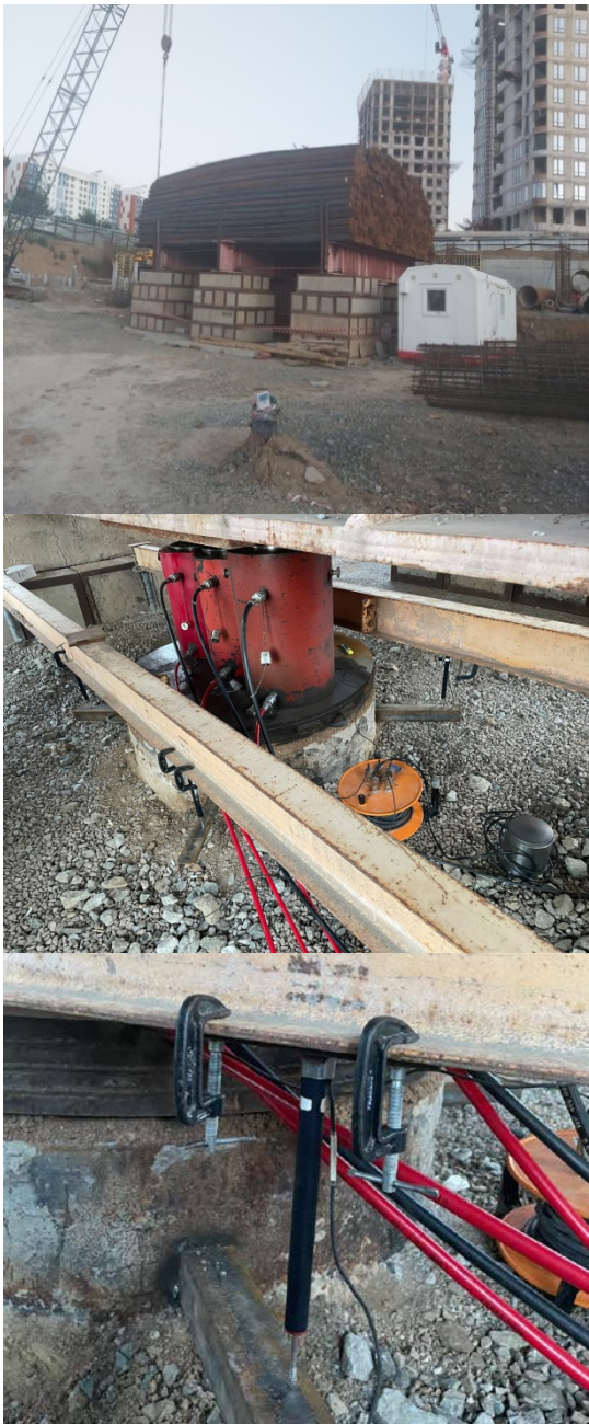
Fig.7 Static load tests boring piles in construction site high-rise building “Diamond”
