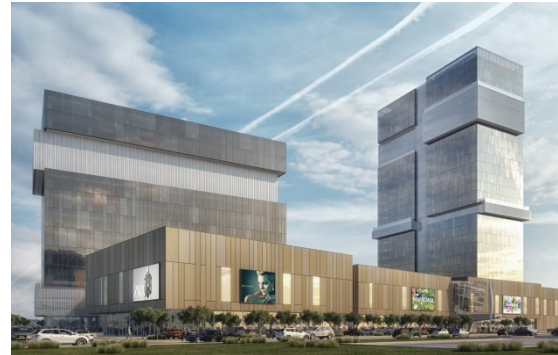
Fig. 2 "Diamond" multi-functional complex
