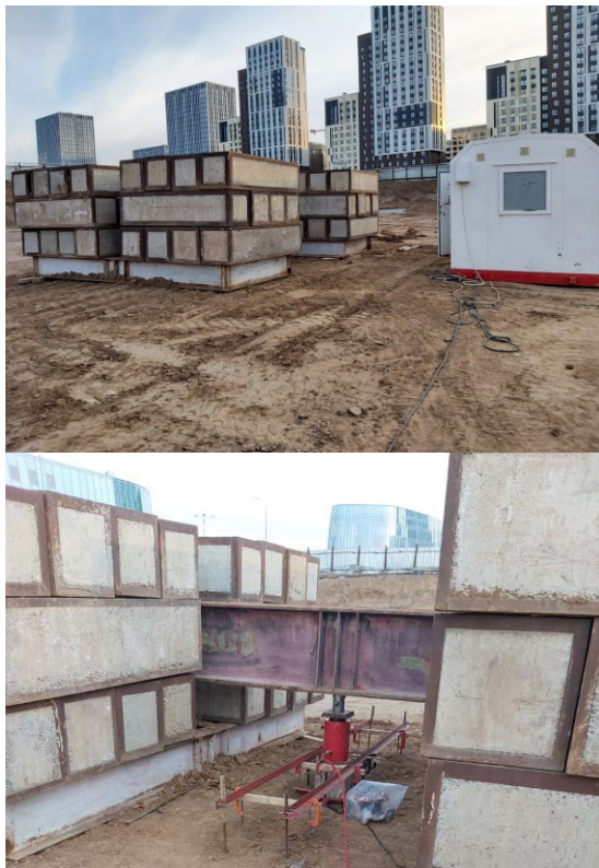
Fig. 5 Driven pile test for static compression
