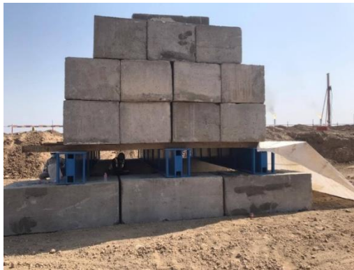
Fig. 4: Pile load test on CFA piles.
