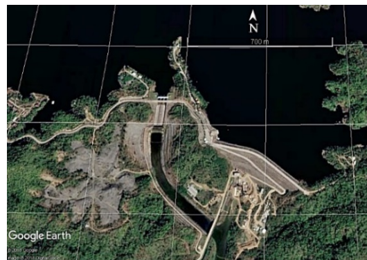
Fig. 2 Kiew Kho Ma Dam and its spillway [16]
