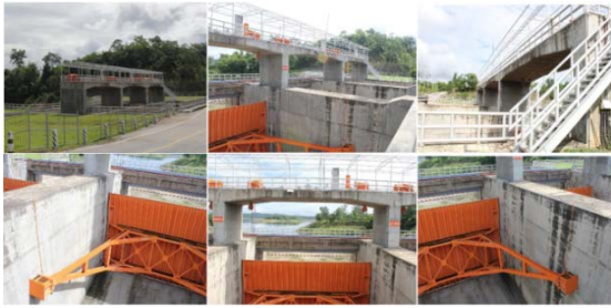
Fig. 3 The Kiew Kho Ma Dam spillway
