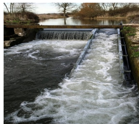
Fig. 3. Ladder-type fish-passing facility
