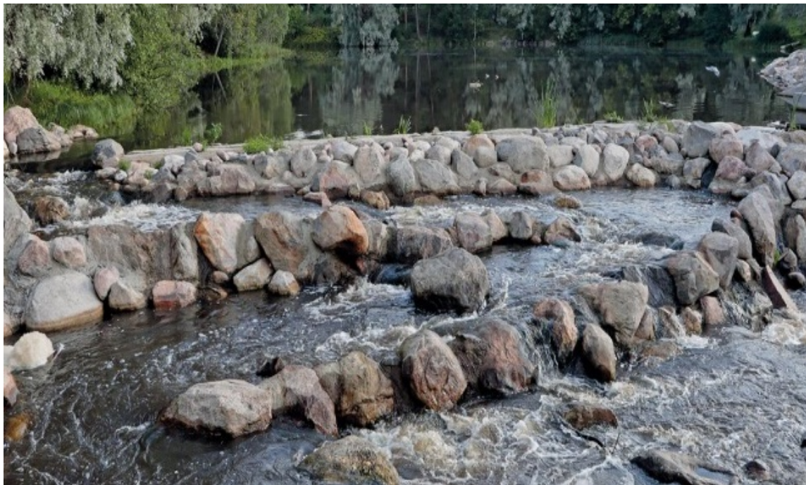
Fig. 2. Improved fish passing structure
