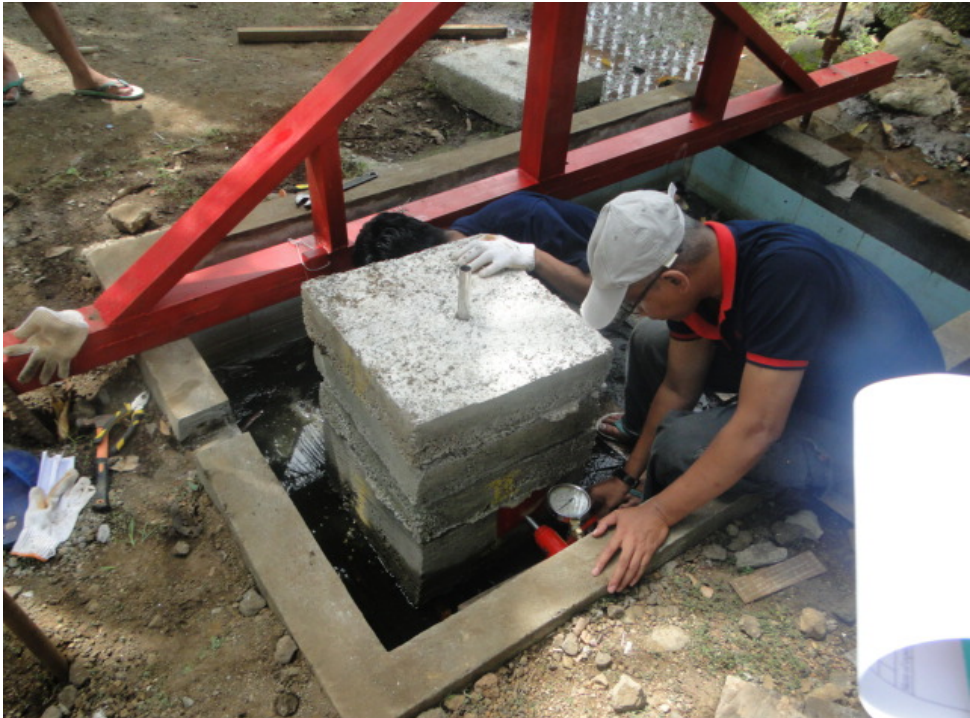
Fig.6 Photo of investigation at the point 1
