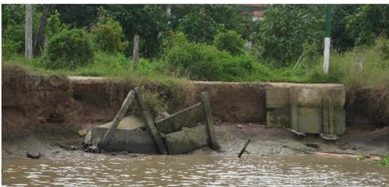
Fig.3 Traditional solution for the stability of Cho Gao canal
