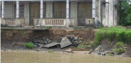
Fig.2 Landslide on both sides of Cho Gao Canal
