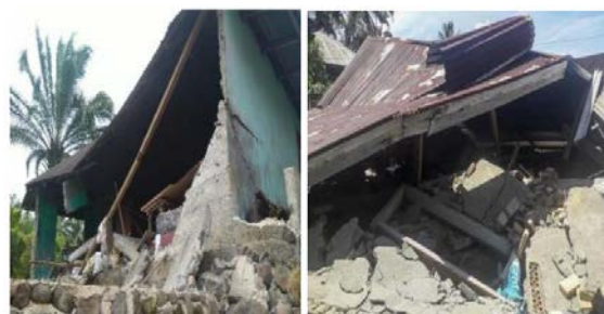
Fig.1 Damage to brick wall houses due to the 2022 West Pasaman earthquake [3]
