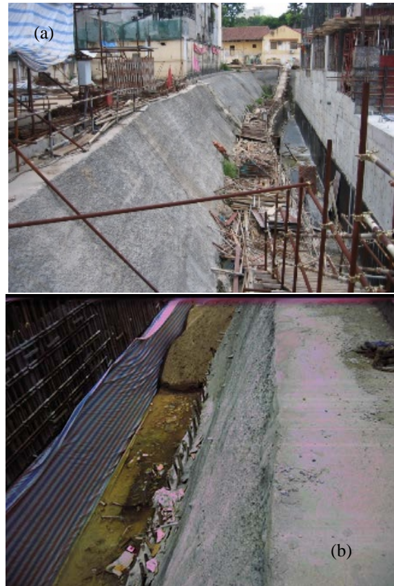
Fig. 3 Excavation slopes at the a) East side and b) North side
