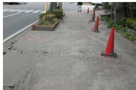
Fig. 1 Liquefaction damage in the 2011 off the Pacific coast of Tohoku Earthquake
