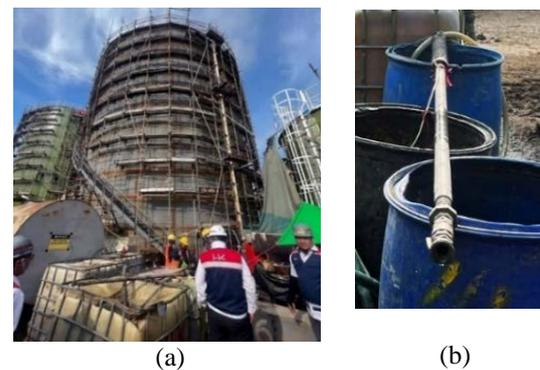
Fig.10 Grouting operation: (a) tank field condition (b) injection pipe
