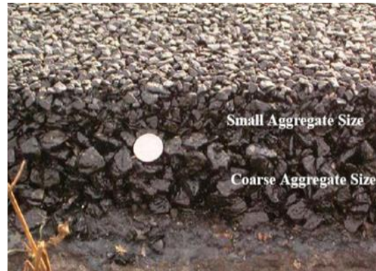
Fig. 2 Porous asphalt mixes' macro- and micro-texture after about ten years of use
