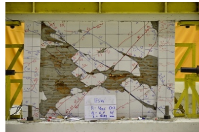
(b) Crack Pattern at R=1/12.5
