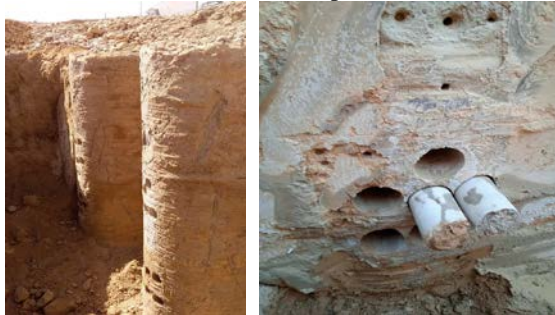
Fig. 1. General view of soil-cement columns
