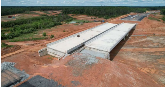
Fig.2 Geofoam technology on the Simpang Indralaya – Prabumulih Zone 6 STA 59 + 425 Toll Road.
