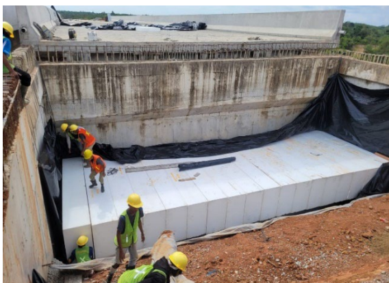
Fig. 12 Construction process of geofoam
