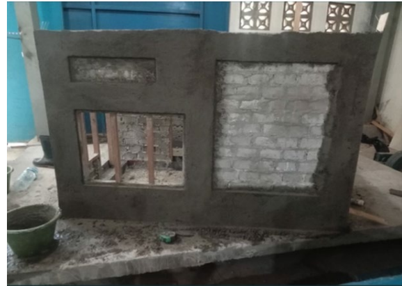
Fig.8 Plastering process of the wall covering the installed woven wire
