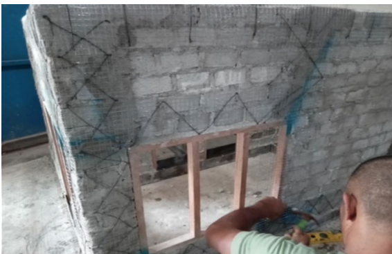
Fig.7 Woven wire installation process
