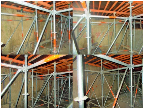
Fig. 15 Photo of B3 after bracing layer 2 removal.
