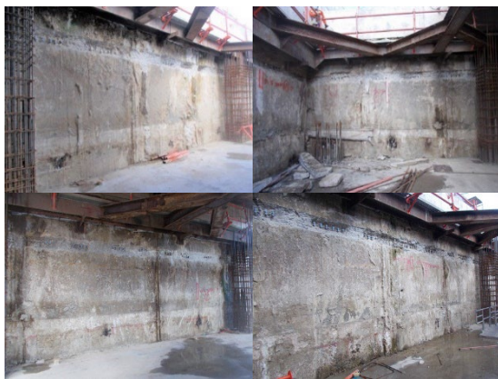
Fig. 16 Image of B2 after bracing layer 2 removal.
