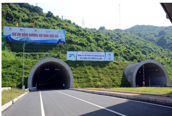
Fig. 1 The DeoCa tunnel.
