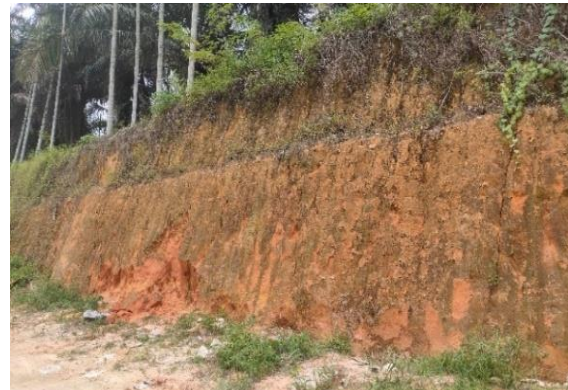
Fig. 1 Condition of the cut slope
