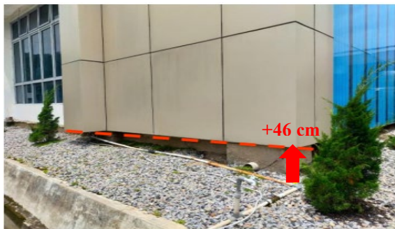
Fig. 2 The right side of the building is lifted
