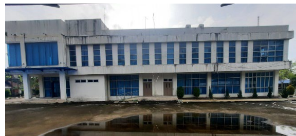
Fig. 1 The RC frame building exposed to differential settlement in Padang City, West Sumatra, Indonesia
