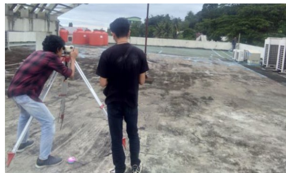
Fig. 6 Geometric measurements on the roof top of the building
