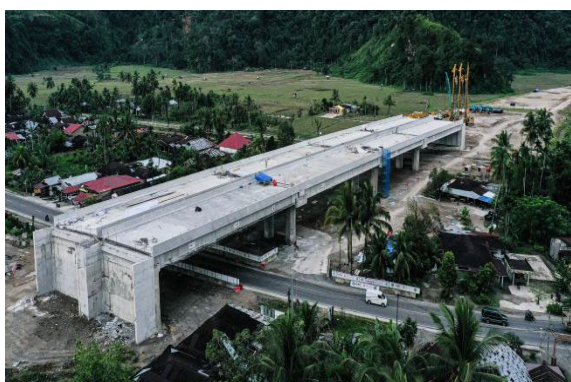
Fig. 2 Prestressed concrete bridge in Padang Pariaman Regency, Indonesia
