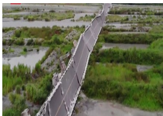
Fig. 1 The Gaoliao Bridge collapsed after a 6.9 M earthquake in Taiwan [2]
