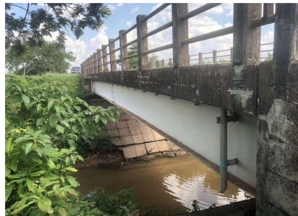
Fig. 2 Steel I-girder Bridge (Bridge No.11)
