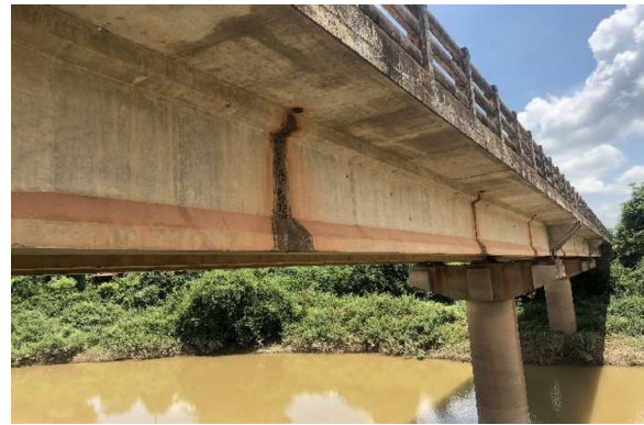
Fig.1 PC I-girder Bridge (Bridge No.5)
