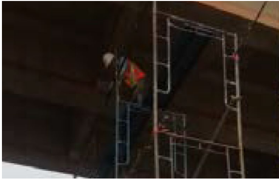
Fig. 6 Instrumentation installation for Bridge No.5
