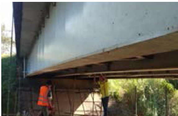
Fig. 7 Instrumentation installation for Bridge No.11
