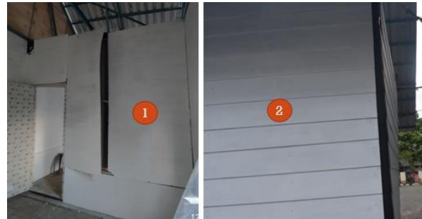
Fig.32 Sheathing damage at 50 kN: a pull-through on one side and the plank are still stable
