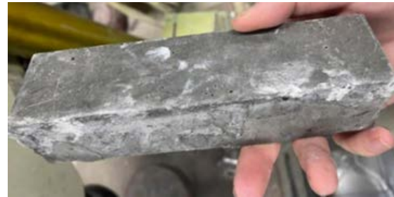
Fig.17 Image of Efflorescence. (FA70)
