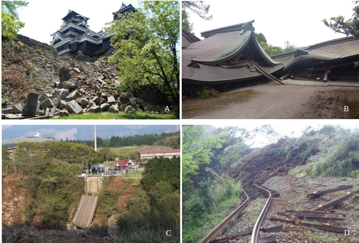
Fig 1 Damage caused by the Kumamoto Earthquake [17,18] ,A: collapsed stone wall of Kumamoto Castle; B: crushed Aso Shrine; C: collapsed Aso Ohashi Bridge; D: uplifted track of Minami-aso Railway Line
