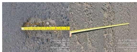
Fig. 2 Manual Road Condition Survey
