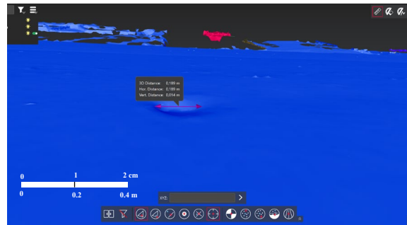
Fig. 8 Road Damage Measurement using TLS
