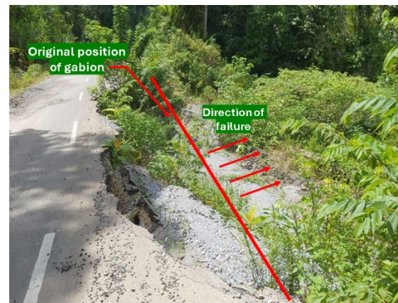
Fig.1 Maligano road section experiences a slope failure.
