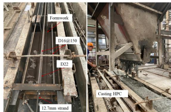
Fig. 5 Casting specimen with HPC
