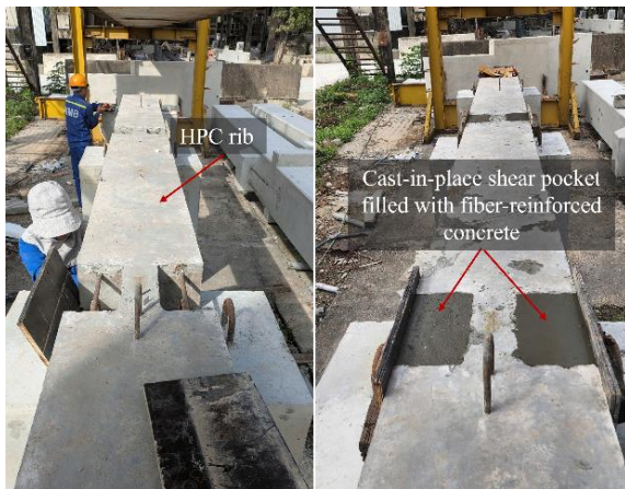
Fig. 7 Filling shear pockets with fiber-reinforced concrete
