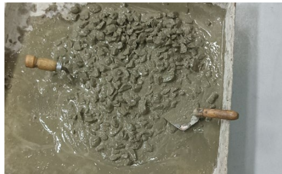
Fig. 1 Mixing of Concrete
