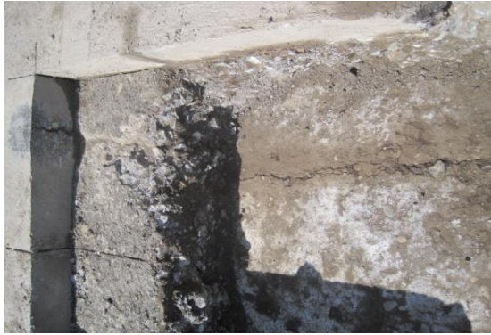
Fig.5 Reflective cracks in the Omsk–Maikapshagai road
