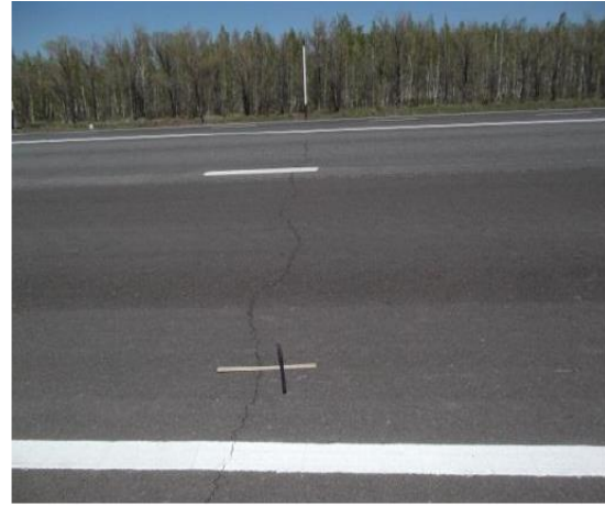
Fig.3 Cracking in the pavement layers of Section of the Omsk-Maikapshagai road.
