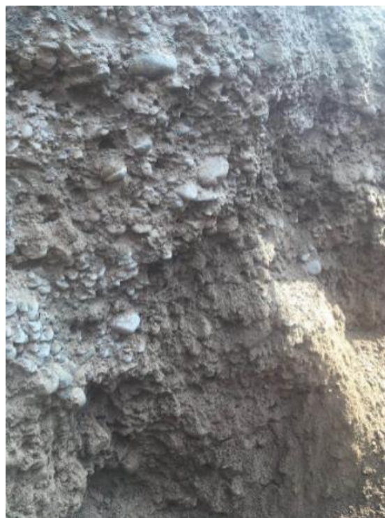
Fig. 3 The stratum exposed in the foundation pit of Yangwan Station
